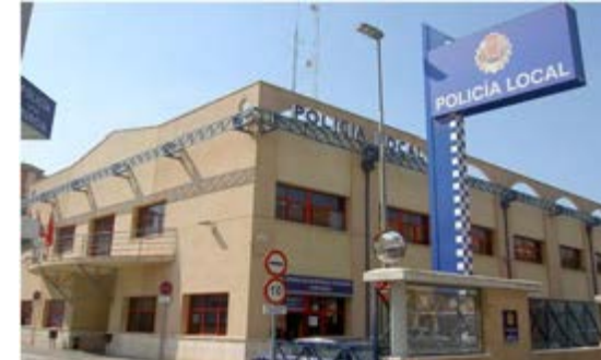
Security Complex of Local Police, Firemen, Traffic and Civil Protection
