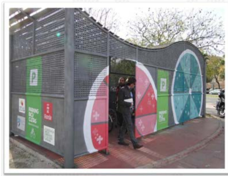
Outside view of a Public bicycle parking
